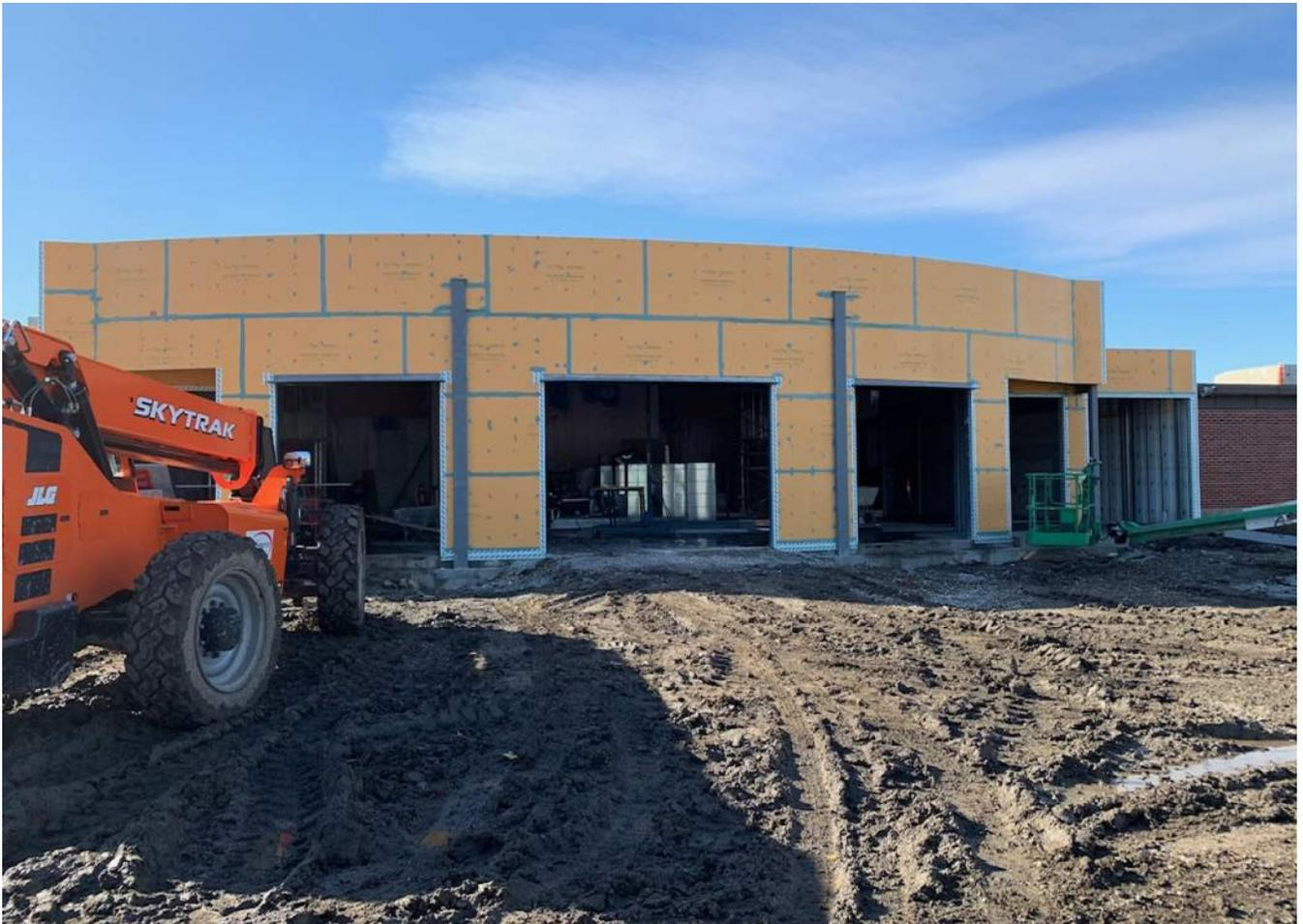
Laying block walls that were removed in order to set new steel.
